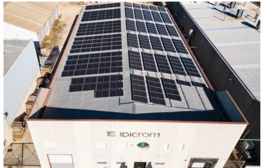
Ibicrom, S.L. / 108,56 kWp / Ibi
